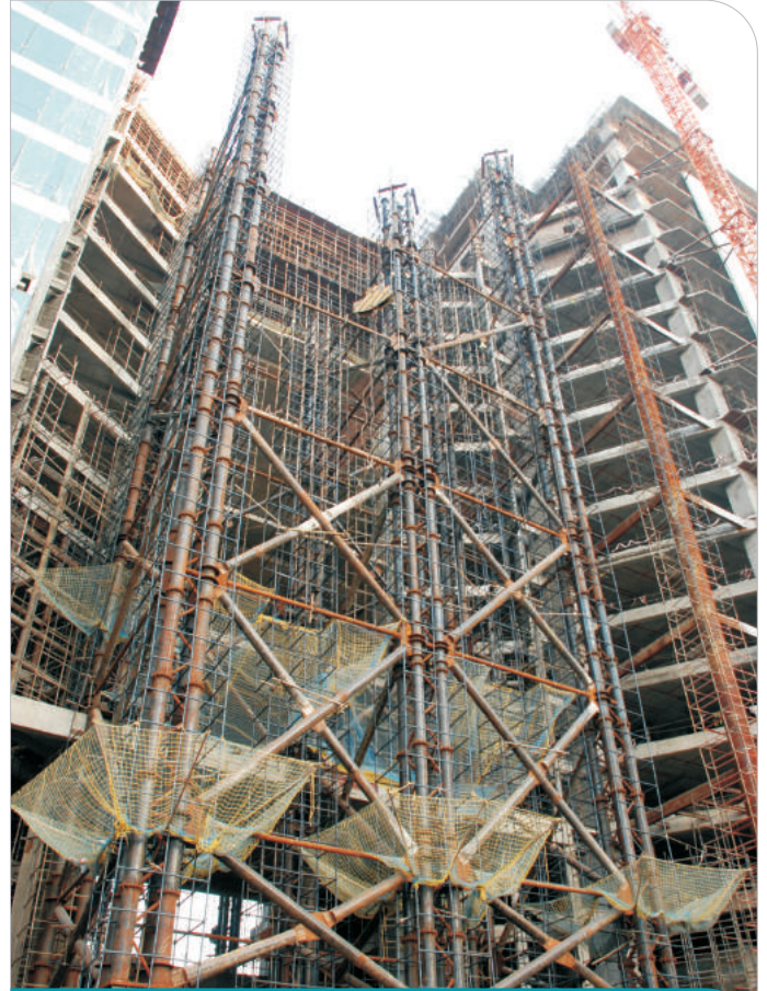
Specially Designed Support System for casting the Suspended Slab at 34th Floor
